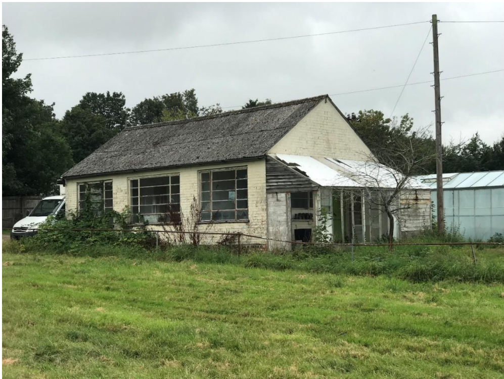
Photo 18: View of a Dilapidated house at the site
