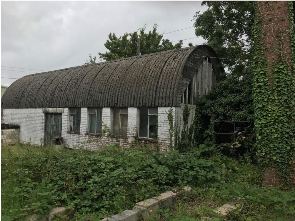
Photo 19: View of 'the Stables' at the site
