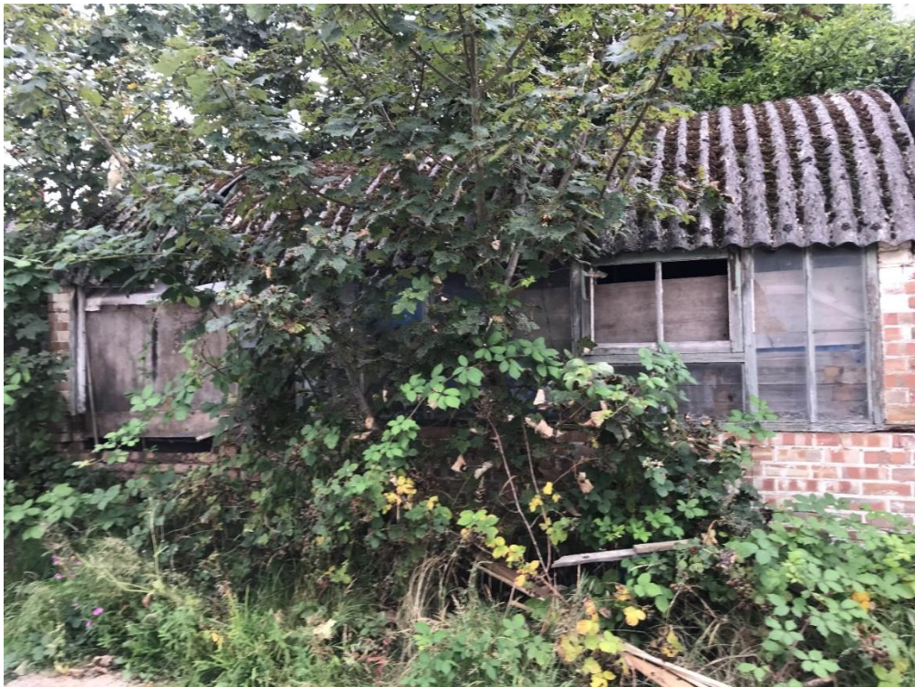
Photo 20: View of 'the Stables' at the site
