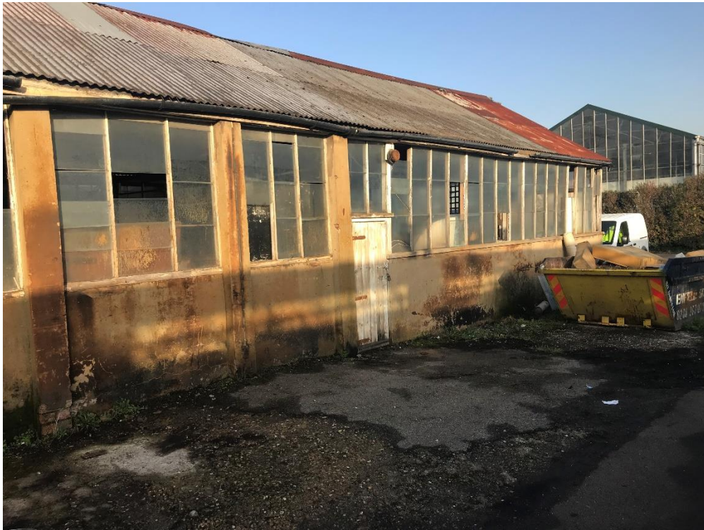
Photo 7: View of a derelict outbuilding at the rear of the site
